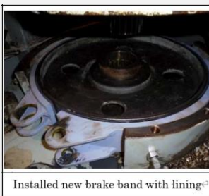
Installed new brake band with lining ©
