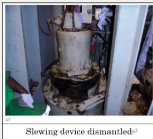
Slewing device dismantled ©
